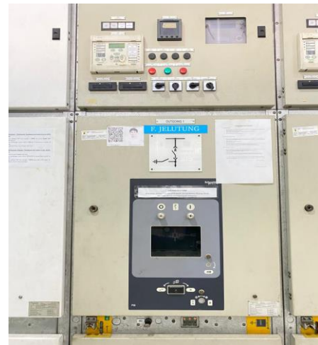
Gambar 12. Panel Feeder Jelutung
